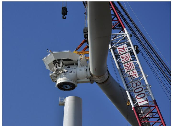
Following some delays in production of the components, the prototype of the SCD 6.0 MW turbine was able to be erected in the Chinese mudflats off Rudong on 3 November 2014. During the installation one of the key benefits of the two-bladed rotor then also became apparent, namely that the entire process lasted **48 minutes**. Its capacity of 6 MW
